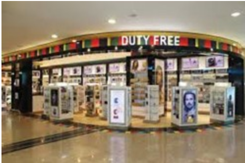
DUTY FREE, CAIRO AIRPORT Fire Alarm & CCTV
