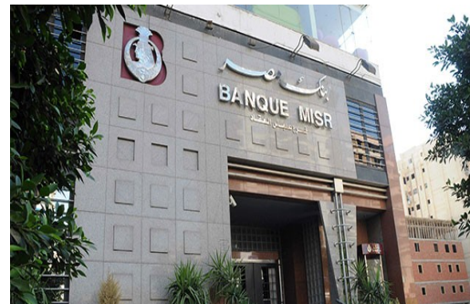
BANK MISR All Light Current Systems
