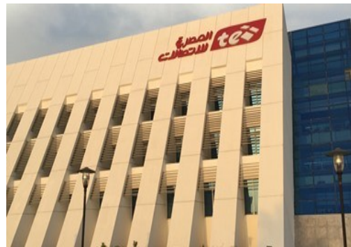
TELECOM EGYPT- Fire Alarm
